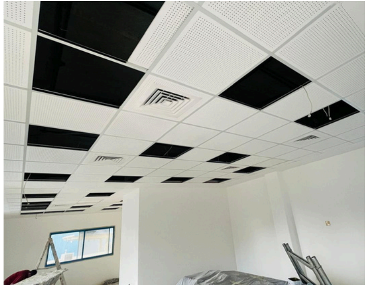
OFFICE RENOVATION PROJECT
