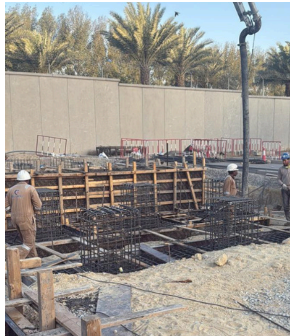
SUBSTATION FOUNDATION WORK
