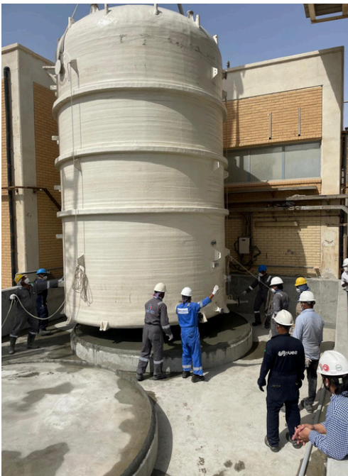
FERRIC CHLORIDE TANK INSTALLATION
