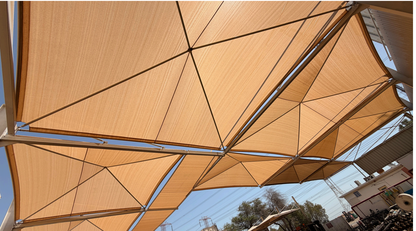
SHADE FABRICATION AND INSTALLATION WORK
