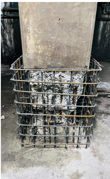
RE PLASTERING AND COLUMN STRENGTHENING
